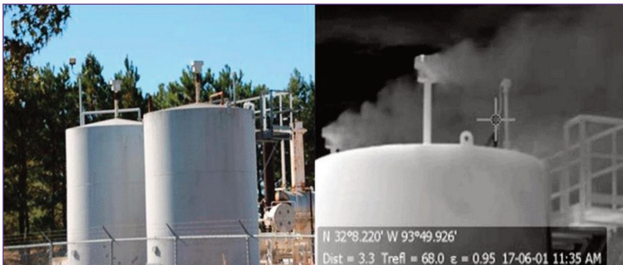
**Figure 2.** Natural gas storage tanks at the Haynesville, Texas, shale fields. Picture on left taken with a normal camera. Picture on right was taken with forward-looking infrared (FLIR) camera tuned to the infrared spectrum of methane, which allows visualization of methane emissions. Photo courtesy of Sharon Wilson. Reprinted from Howarth (2019).<sup>3</sup>
