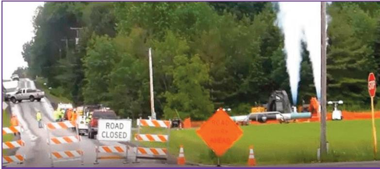
**Figure 3.** Blowdown for maintenance of a natural gas pipeline in Yates County, New York. Methane is an invisible gas, but the cooling from the rapid blowdown condenses water vapor, leading to the obvious cloud. Photo courtesy of Jack Ossont. Reprinted from Howarth (2019).<sup>3</sup>
